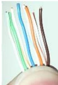
3. Untwist the pairs so they will lay flat between your fingers. The white piece of thread can be cut off even with the jacket and disposed (see Warnings). For easier handling, cut the wires so that they are 3/4" (19 mm) long from the base of the jacket and even in length.
